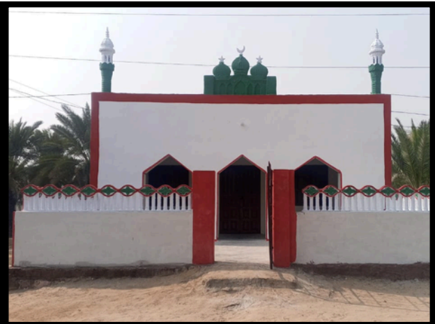
Renovation of Mosque at Saleh Pat Village , Sukkur
